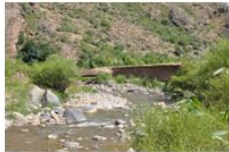
Pictures 2. Eroded bank of Yeghgis River in Shatin community.
