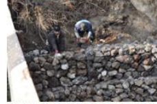
Picture 5. Construction of gabions on Yeghgis River, Shatin community.
