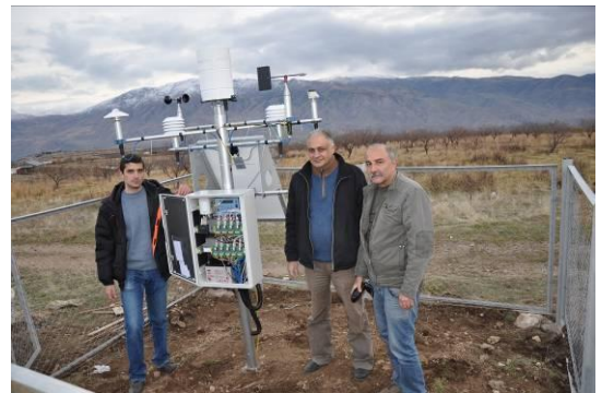
Figure 2. Hydromet Service specialists during the installation process.
