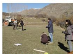
Picture 5. Construction preparatory work.
