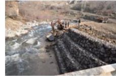
Picture 4. Construction of gabions on Yeghgis River, Shatin community.
