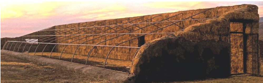
Figure 5. Passive Solar Greenhouse, construction process.
