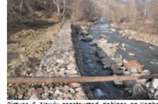
Picture 6. Newly constructed gabions on Yeghgis River, Shatin community.
