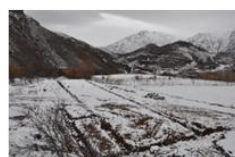
Picture 6. PSG construction site in November, 2014.
